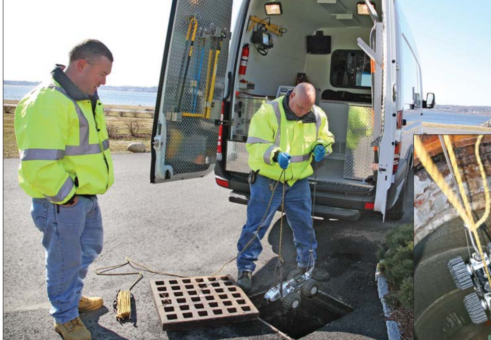
Mat Solitro (left) and John Hannon deploy the crawler to televise a line.
