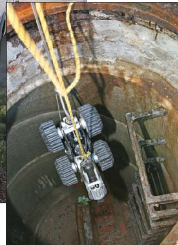
A single operator can deploy the camera and crawler into manholes.
