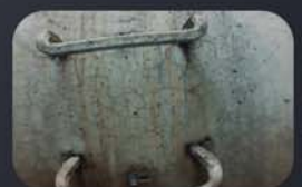
Wide view in manholes
