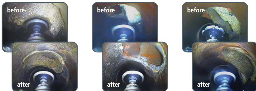
HydroCut eliminates the burrs gouges and tearing (shown here) left by pneumatic cutters.
